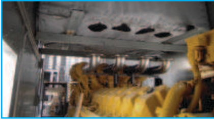
GenAcc's AirClarity system equipped on a Caterpillar C-175 engine.
